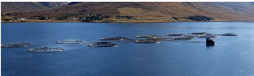
Photo 2: Loch Ainort, Skye: Typical fish farm arrangement of two rows of six pens within a submerged mooring grid and a feed-barge.
